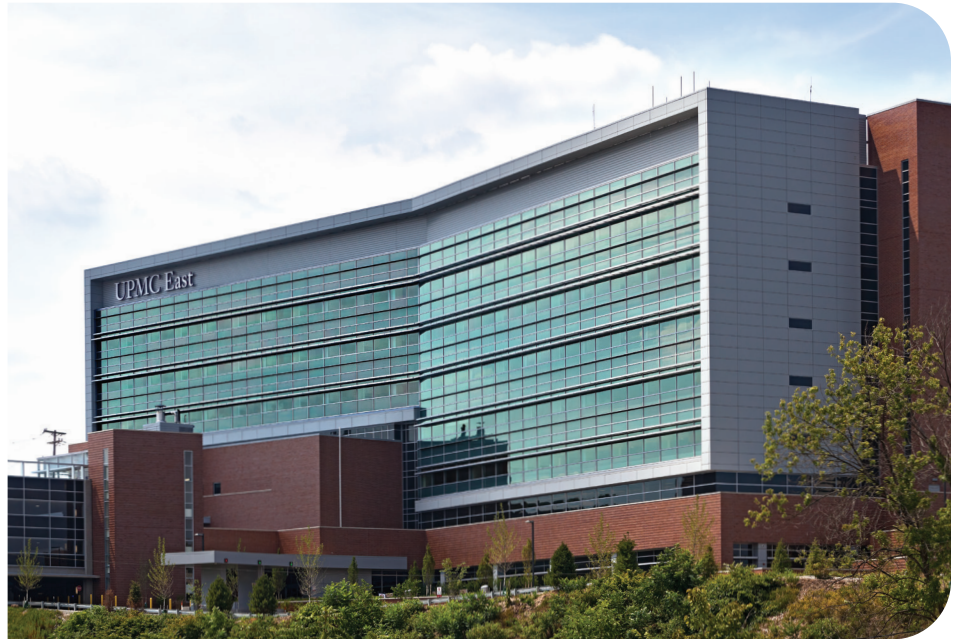
Constructing UPMC East on an east-west axis lowered the hospital’s solar heat gain by 17 percent. Solarban ® 70 and Solarban ® 60 glasses are part of a super-insulating building envelope that provided the performance and aesthetics the owners desired.
